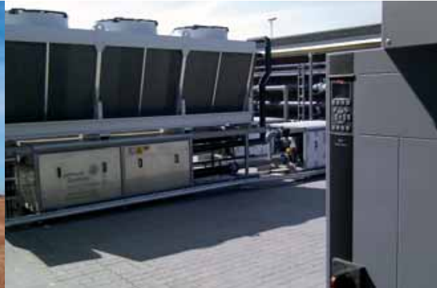
Two VLT® Advanced Active Filters for HVAC installed at a hospital to ensure a stable supply for vital equipment.
