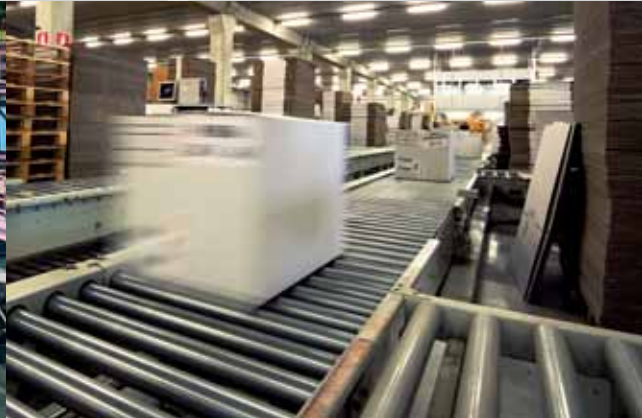
Six cost optimized VLT® 12-pulse drives incl. transformer installed at facility for material handling.
