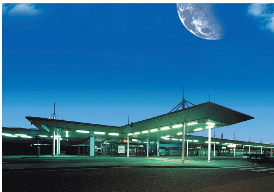
Belfast International Airport handles over 5,000,000 passengers per year.
