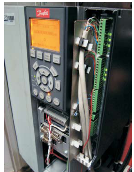
SyncPos cards installed on VLT® Automation Drive.
