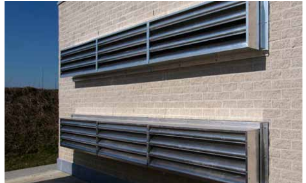
There is a low level of noise generation outside the building because of noise absorbing exhaust ducts.
