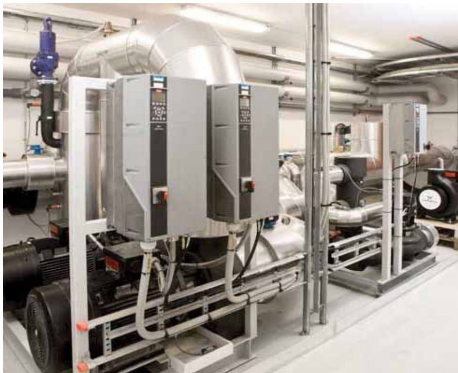
VLT® HVAC Drive FC 102, 37 kW, IP55 enclosure installed on the central pump.
