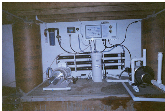
First USA APP pump installation
