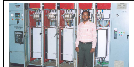
VLT 6100 (75 kW) for SCHW pumps installed in an MCC shown along side Mr. PG Patil. Picture below shows their pump layout.
