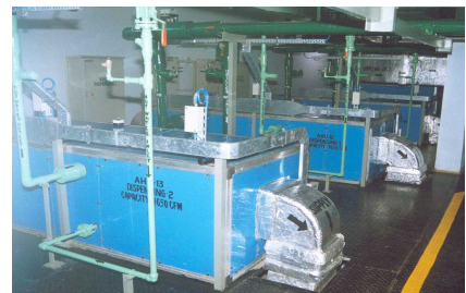
AHU with Danfoss VLT 6000 in operation along side Mr. BB Shah. Inset shows the VLT 6000 inside the panel. Bottom picture shows their typical service floor layout
